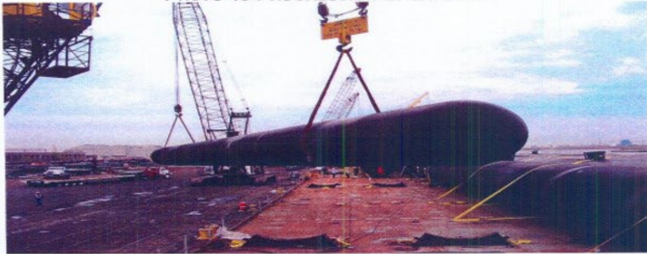
PHOTO 45 PROGRESSION OF LOADING
